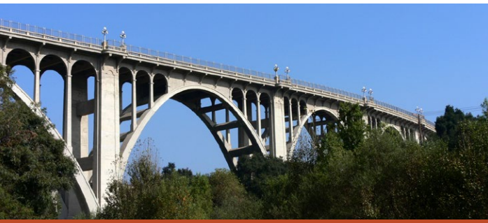
COLORADO STREET BRIDGE
