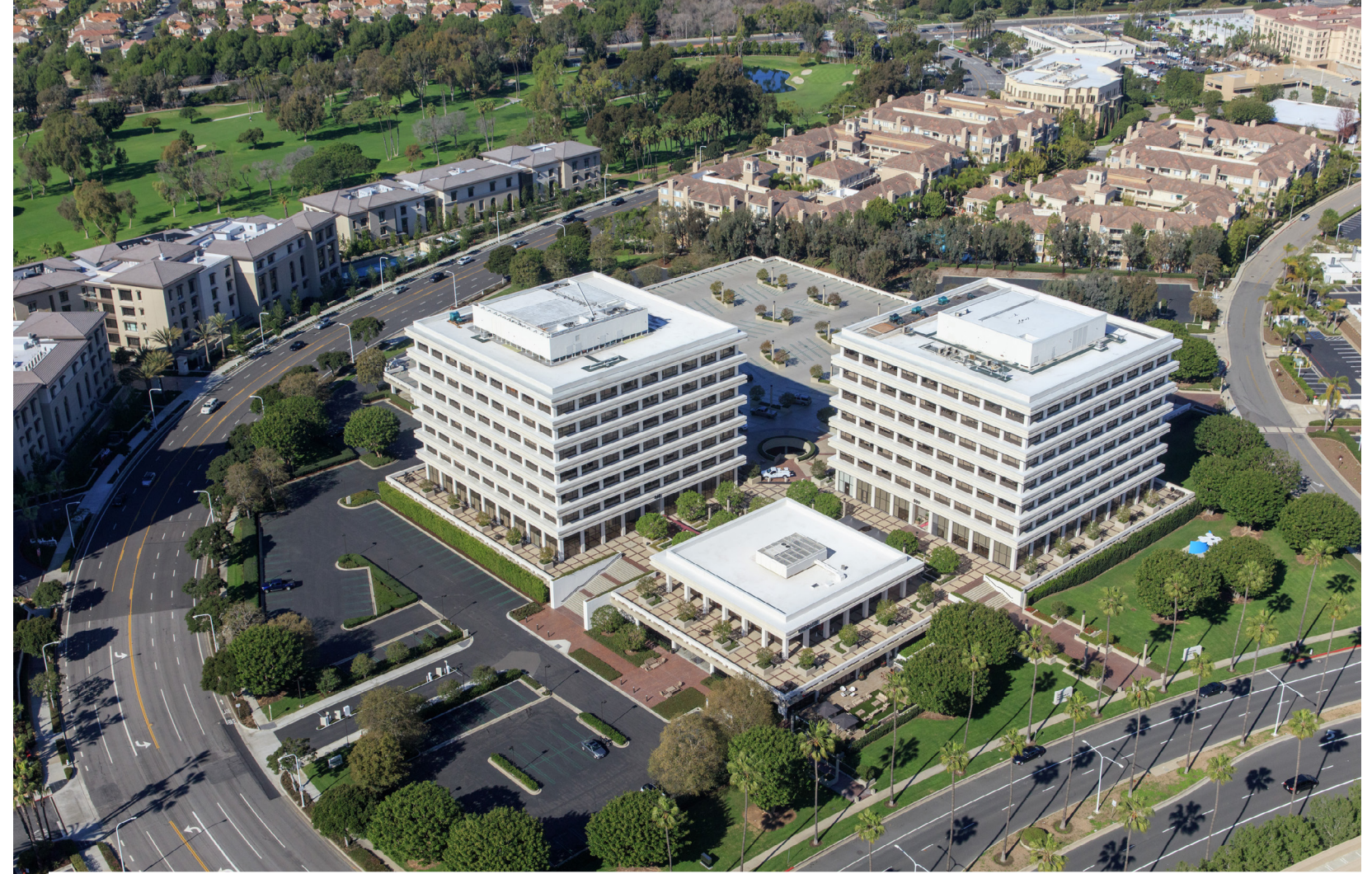
800 BLOCK: 800, 840, 860 AND 880 NEWPORT CENTER DRIVE
